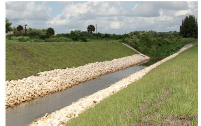
To correct the failed slopes and provide protection into the future, the banks were first re-graded, then armoured with rip rap at the toe and HPTRM up to the head. The high flow velocity of the channel necessitated increased pullout resistance of securing methods. As a result, the Gripple Terra-Lock™ System was chosen to secure the HPTRM and provide an additional factor of safety. This system has subsequently been proven to be effective, holding under a 203 mm (8") rainfall event.
