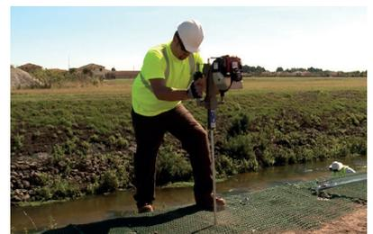
The sandy soil meant that the TLA-2 anchors were easily drivable to a depth of 1.2 - 1.8 m (4 - 6 ft) and comfortably met the required 70 kg (150 lb) pullout resistance. The installation process was eased through use of Gripple installation tools including; GPD, JackJaw®, Drive Rod and Wire Cutters. On this site the JackJaw® was of particular importance, allowing for straightforward extraction of the Drive Rod.
